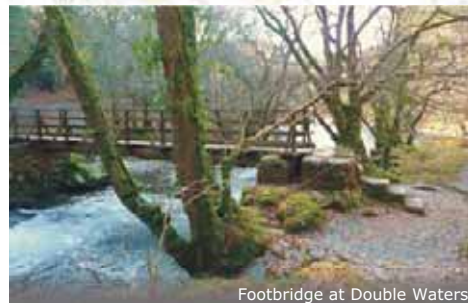
Footbridge at Double Waters
